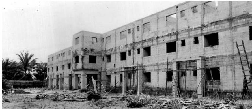
Owerri Grand Hostel, Gearing for Completion.
